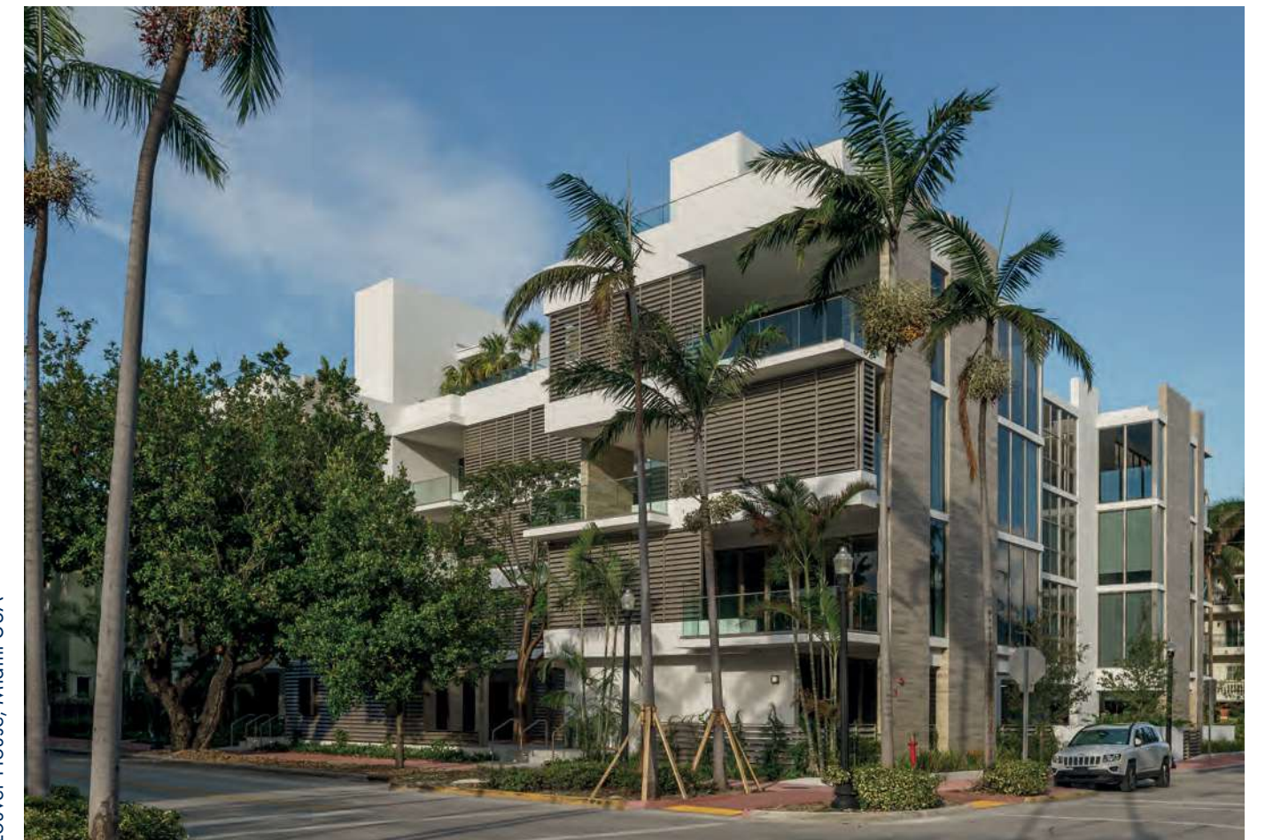
Louver House, Miami USA
